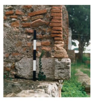
Fig. 11. Caseggiato del Larario, 1 ix 3, provides a fine example of a moulded pilaster base (photo author).
